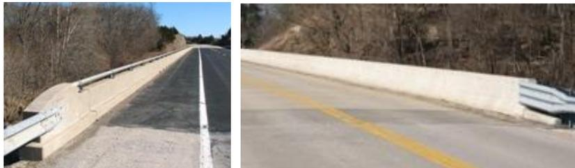
39. **Guardrail End** - May be painted a warning color and may include a breakaway or redirection design feature not to be confused with an [impact attenuator/crash cushion](#).
