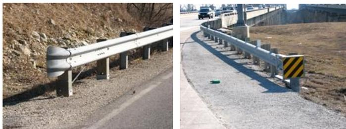
40. **Other Traffic Barrier** - Longitudinal barriers other than guardrails, concrete traffic barriers, or cable barriers. They may be composed of material such as wood or rock.
